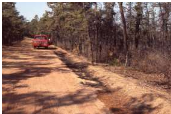
FIRE IGNITION ATTRIBUTED to PARKED VEHICLE on SHOULDER of ROAD with PINE-NEEDLE LITTER, RED ROAD, PENN FOREST
